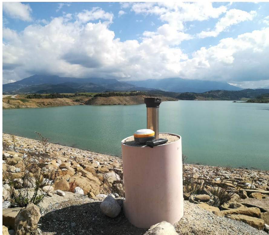
Figure 3. A typical example of performing static GNSS measurements on permanent pillar located on the crest of Asteri dam, Western Greece.
