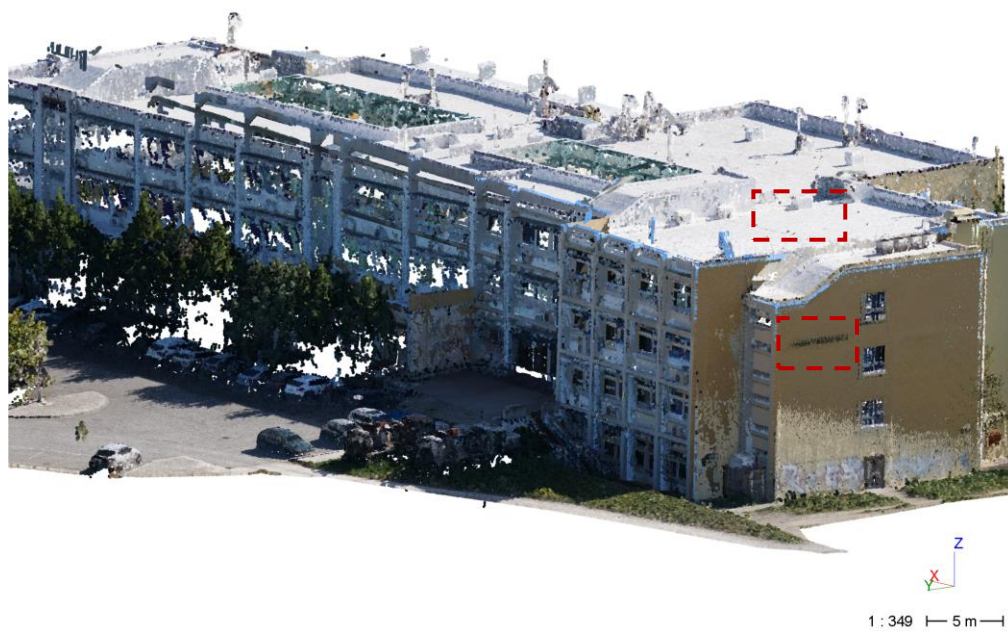
Figure 11. Fused point cloud of the Department of Geology at the University of Patras (oblique view).
