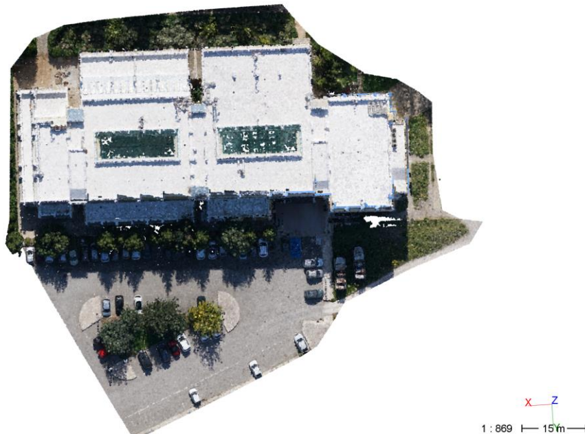
Figure 5. UAV point cloud of the Department of Geology at the University of Patras (top view).
