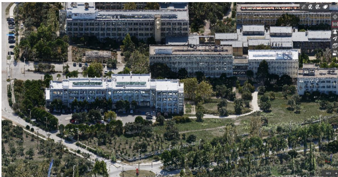
Figure 4. 3D view of the University Campus. A dense point cloud was produced by the Vtol UAV imagery.
