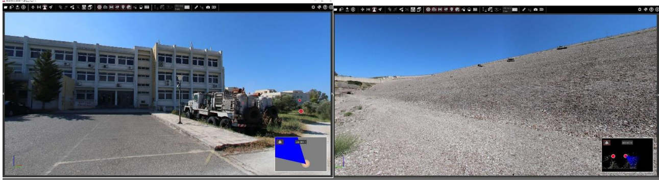
Figure 3. (a) 3D representation of the Geology Department building. (b) 3D representation of the Asteri Dam. Both point clouds are captured with Leica P50 scanner.
